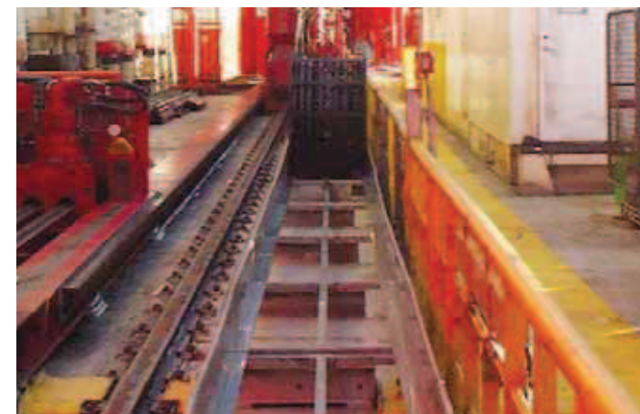
System E4 with extension links -long travel application onboard West Navigator (Norway)
